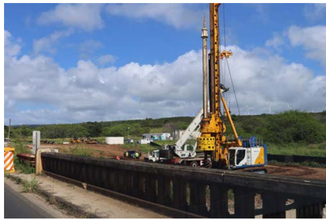
State DOT project contractor Goodfellow Brothers drilling a "test Shaft" Photo: Betty Depolito
