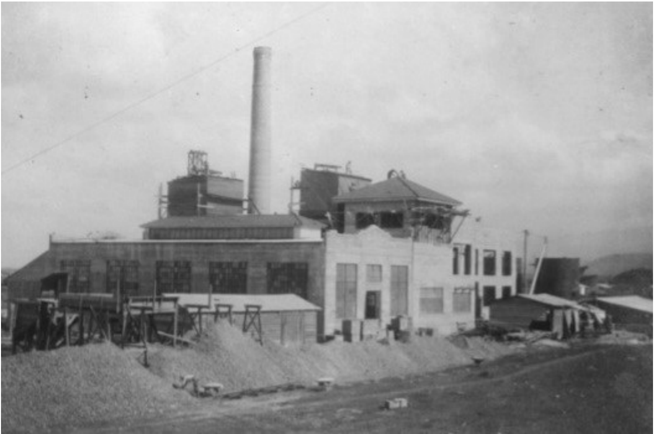
Marconi Wireless Telegraph Station, Operating Building, Circa 1910.
