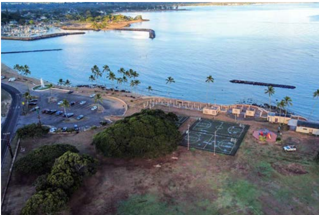
Bird's eye view of park showing what's left of the original structure. Photo: Mike Fritz
