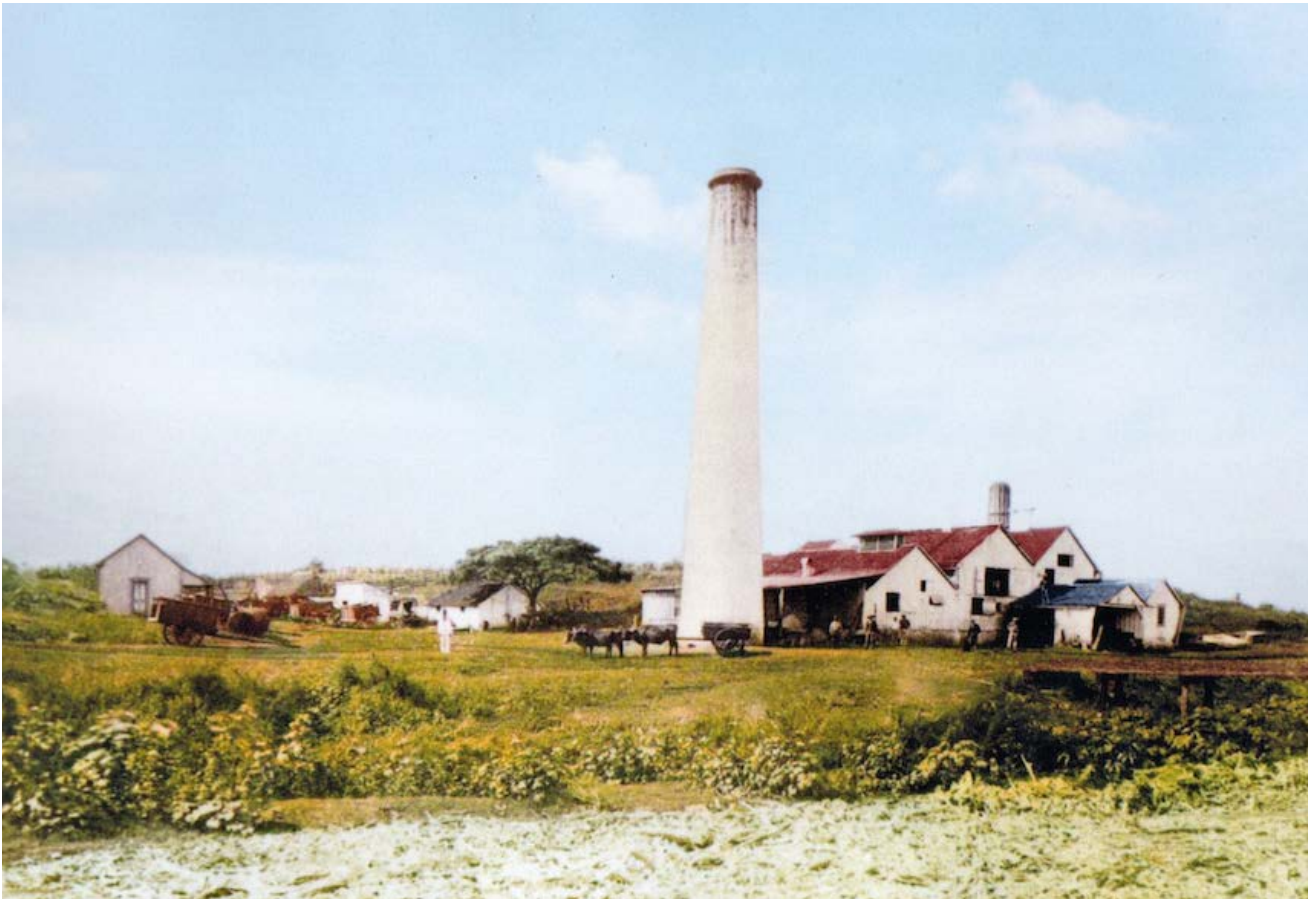
1890's Halstead Mill, Waialua, Hawaii Photo Courtesy of North Shore Photography and Hawaii State Archives
