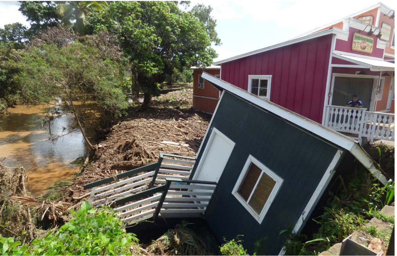
Flooding and damages in Hale'iwa Town Photo: Mike Fritz
