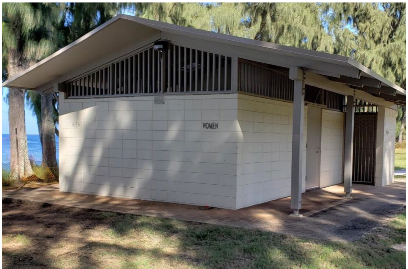
Three Tables restrooms renovations completed. Photo: City and County of Honolulu
