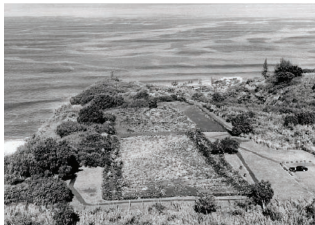
1970's, view overlooking the Heiau
